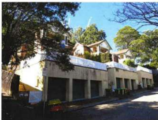
Photo A2– View of Existing Dual Occupancies West of the Site at 1-5 James Street
