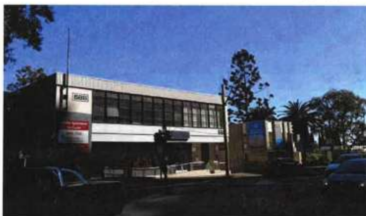
Photo A1 – View of Site Looking Northwest from the Pacific Highway
