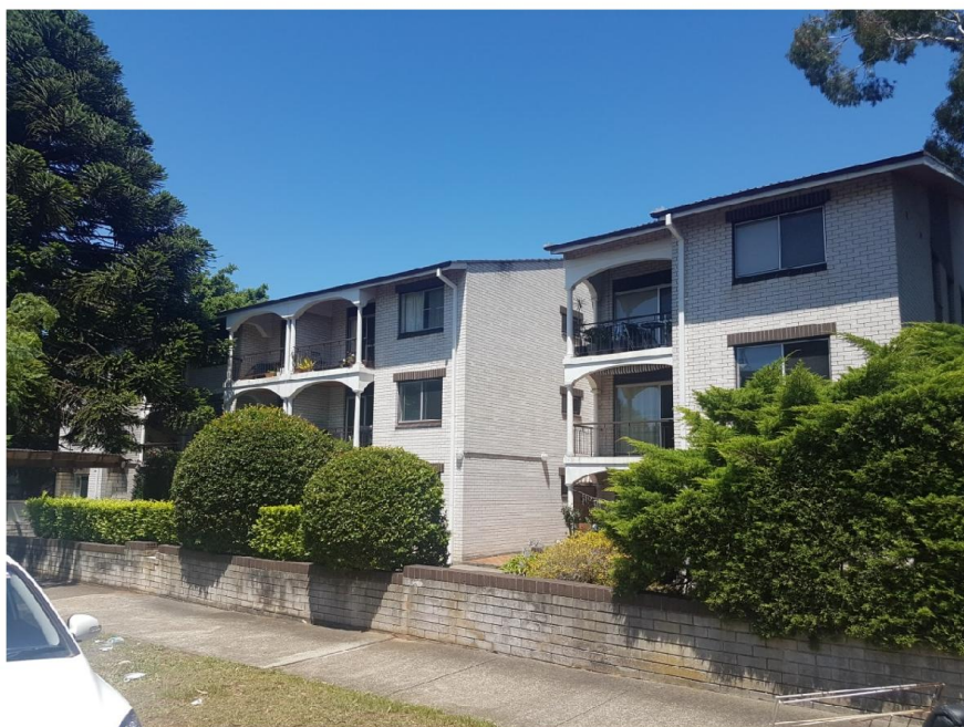
Images 1A and 1B: 2-6 Bowen Street taken at 11:45am in summer, showing self-shadowing due to built form and surrounding vegetation.
